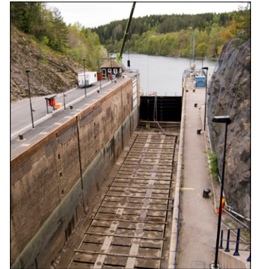
Every lock chamber is 90 metres long, 13-18 m deep and 13 m wide.
