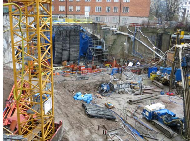
The railway tunnel in the bedrock is opening up behind what once was a small lake, now undergoing ground reinforcement.
