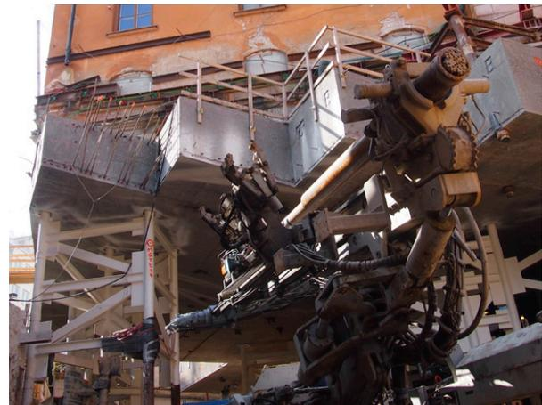
Wassara W150 hammer, ready for casing advancing under the building. The tunnel roof is clearly visible here. (Photo courtesy of Bilfinger Spezialtiefbau)
